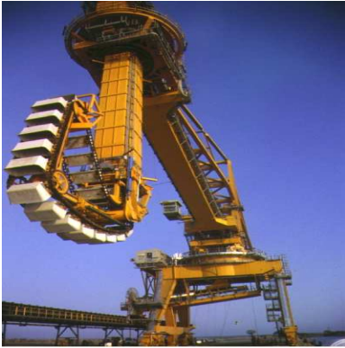
The continuous ship unloader on the wharf
