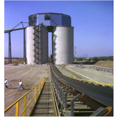
Coal storage silos
