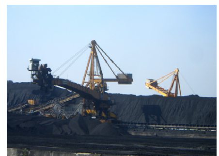
General view of the coal storage area
