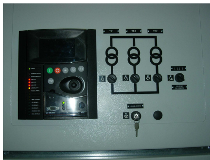
Detail of Protection on Metal Clad
