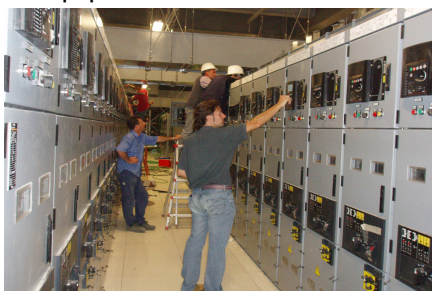
LV-MV panels w/GE-F650 protection
