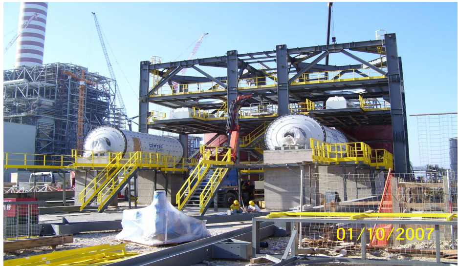
Limestone Milling system - General view of the plant during construction
