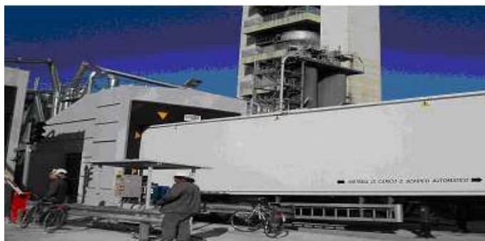
Automatic truck unloading
