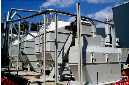
RDF Plant in a cementery
