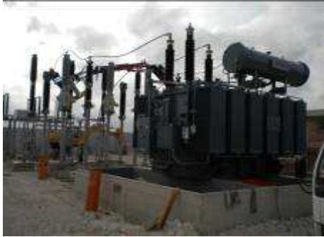
Transformer 150/20kV
