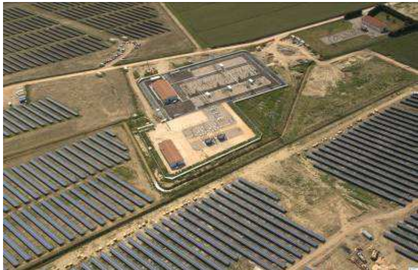
Aerial view of the Producer and TERNA double busbar station
