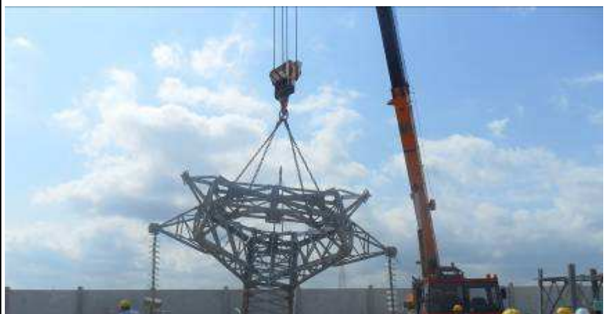
Erection of the pylon (palo gatto)
