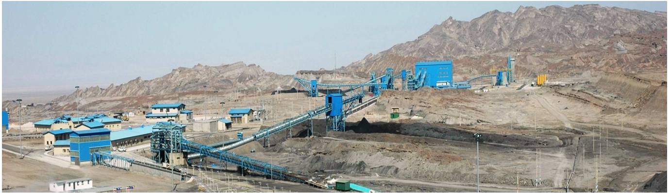
General View of the Coal Handling and Treatment plant
