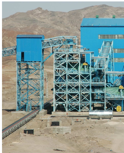
View of the main belt conveyors
