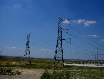
Entrance to the station: Larino FG line
