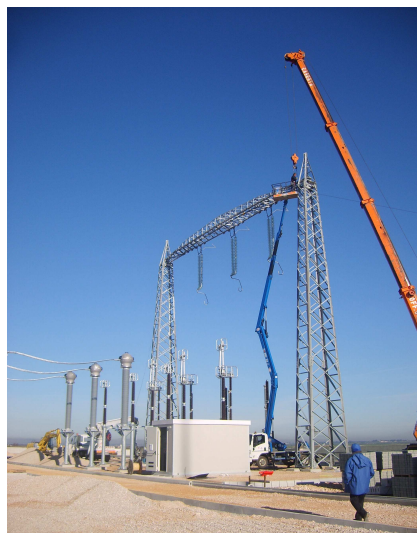
Erection of OHL portal
