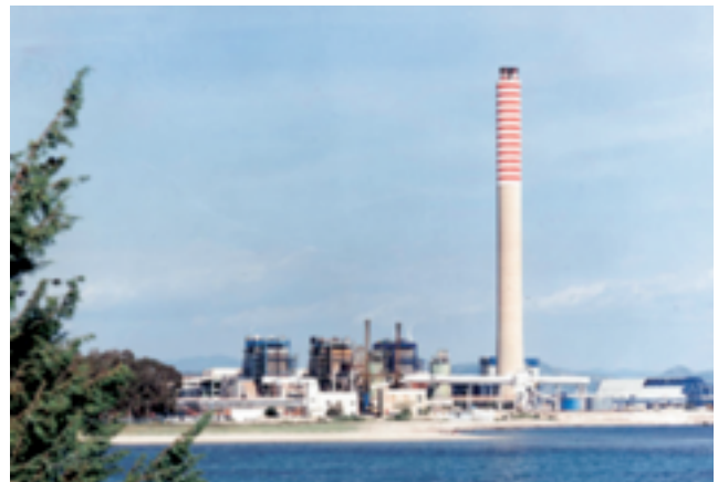
Fig. 1 - Sulcis Power Plant
