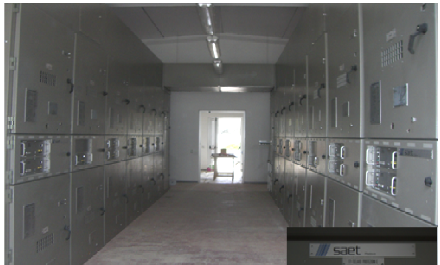
Double Stage Arrangement Panel with 20 kV Distribution
