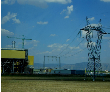
View of the ENPLUS Power Plant
