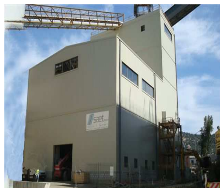
Limestone Milling building
