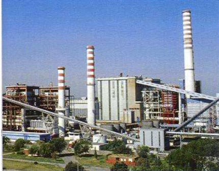
General view of the Thermo Power Plant
