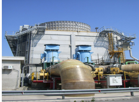
Circulation pumps for water
