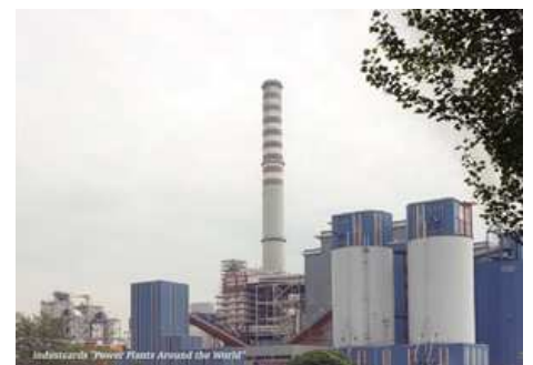
View of the ENEL Fusina thermo power
